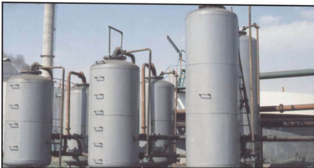
Tertiary system to streams 100 M 3 /hr. each Power sand filter followed by plant based activated carbon & polishing unit comprising high grade anthracite and activated carbon
