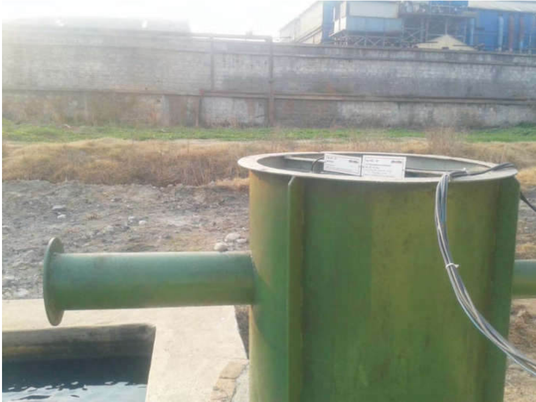
Treated Water outlet Tank
