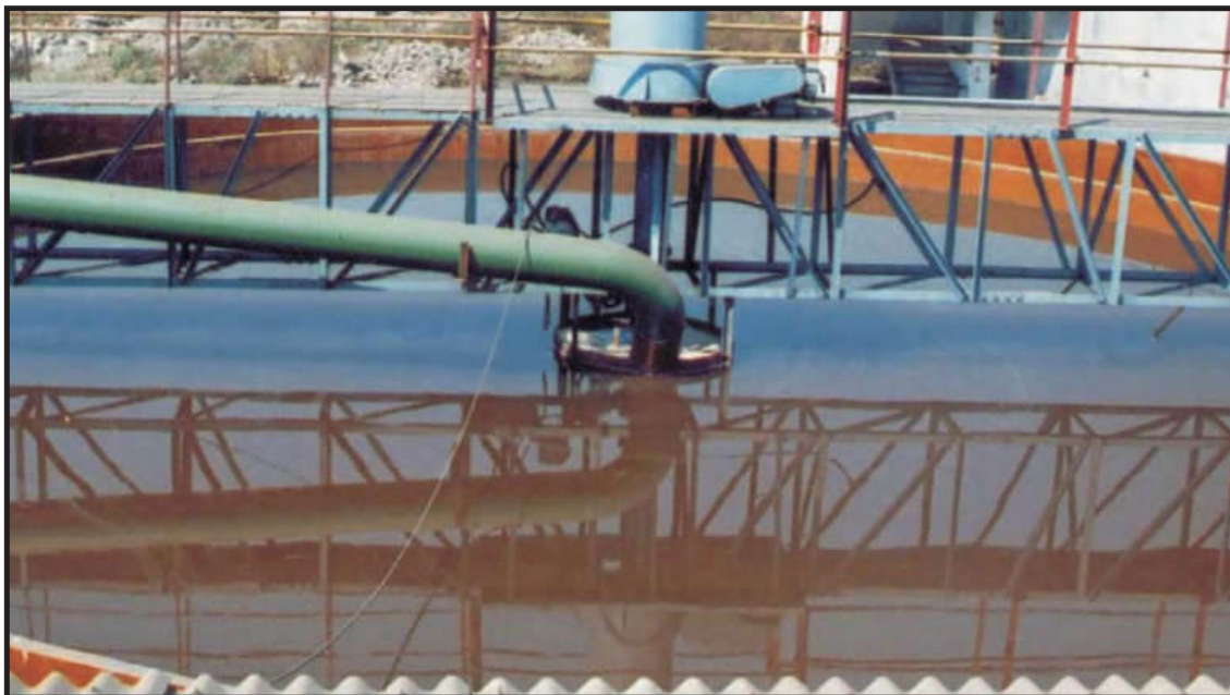
Secondary clarifier new stream
