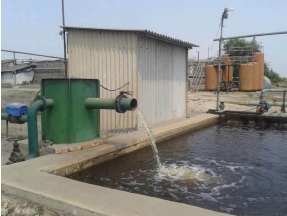
Treated Water Outlet
