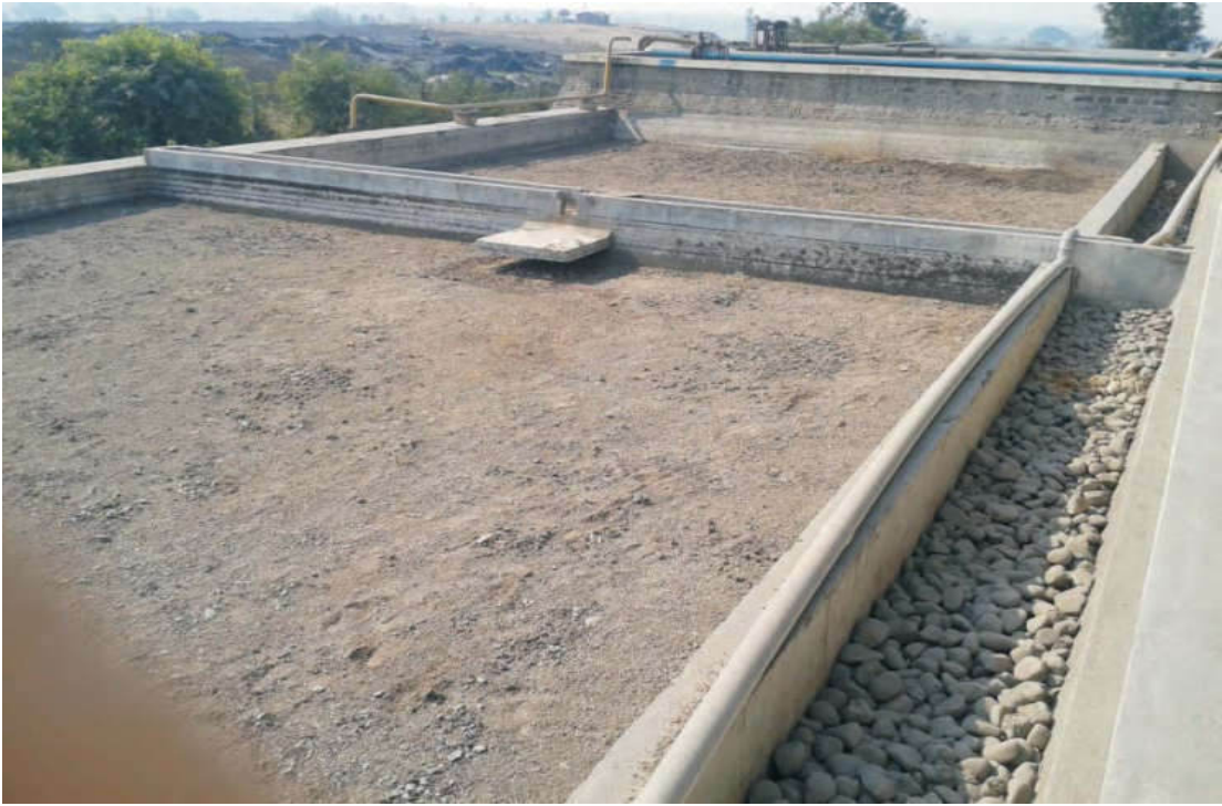
Sludge Drying Bed
