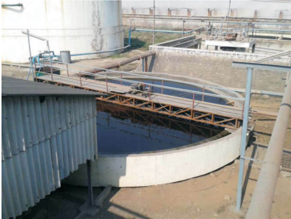
Secondary clarifier old stream
