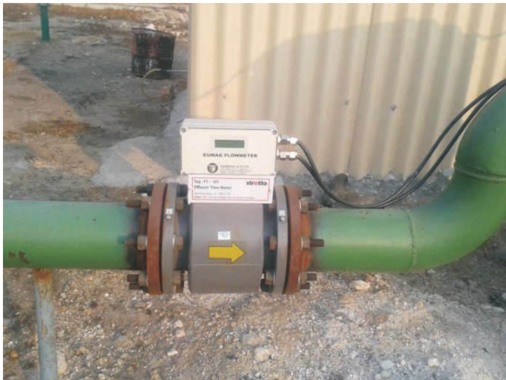
Flow meter for outlet Treated Water
