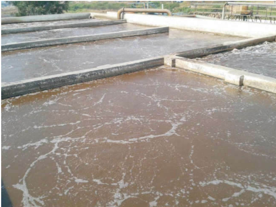
New diffuse aeration tank
