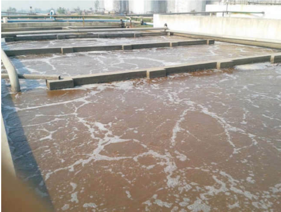
Old diffuse aeration tank
